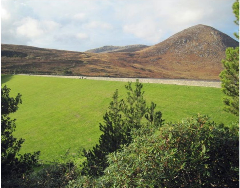
Figure 3: Silent Valley embankment dam in Northern Ireland (1923-1932); Engineer F W McCullough.
