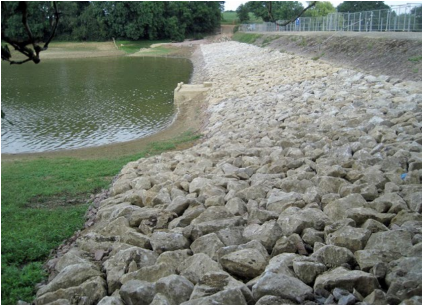
Figure 9: Wave protection pitching at Bosley Reservoir, Cheshire (top); rip-rap at Sulby Reservoir, Northamptonshire (bottom)
