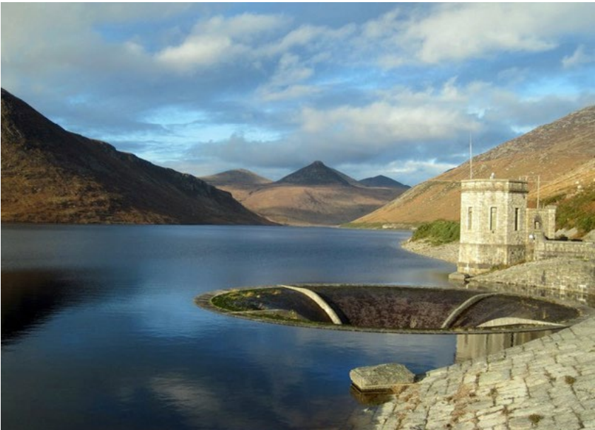
Figure 7: Spillways, Winterburn Reservoir (top); Silent Valley (bottom)
