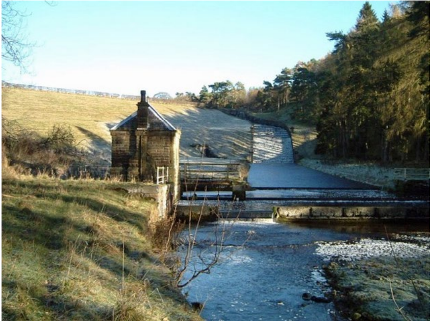
Figure 2: Winterburn Reservoir, near Gargrave, Yorkshire; Engineers Henry Rofe and Edward Filliter.
