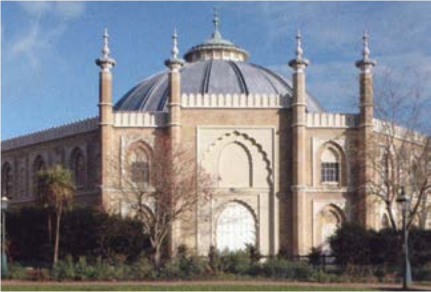
Figure 4. Porden's stable block
