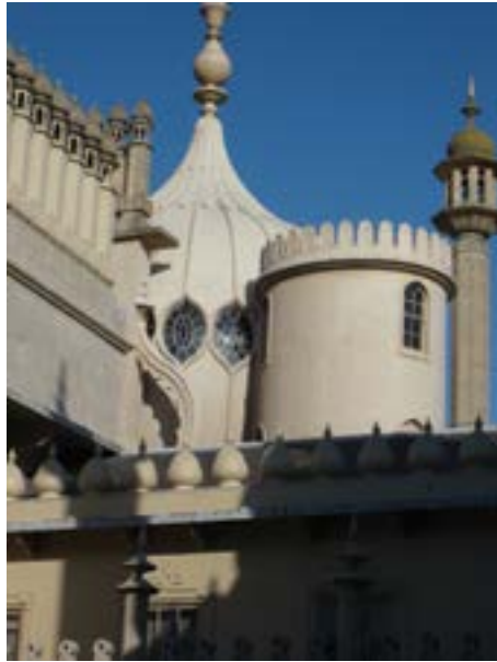
Figure 7: Complexity of roof line.
